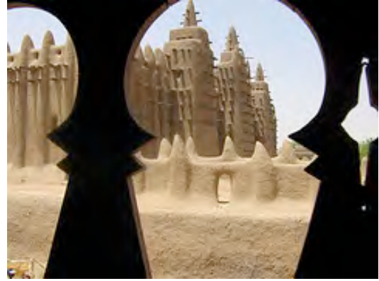
Fig 1.4 Djenne Mosque, Mali
